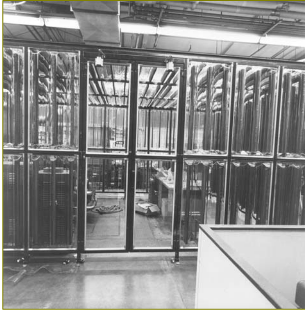
Electronics Manufacturer Needed To Reduce Noise And Provide A Class 10,000 Room Within A Class 100,000 Environment
