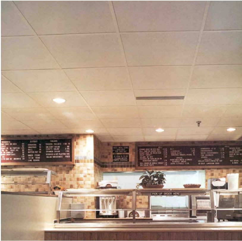
Good Acoustics and sanitary conditions are critical in food prep and point of sale areas.
