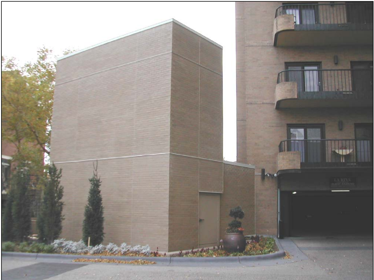
Cooling Tower with Aeroacoustic Enclosure
