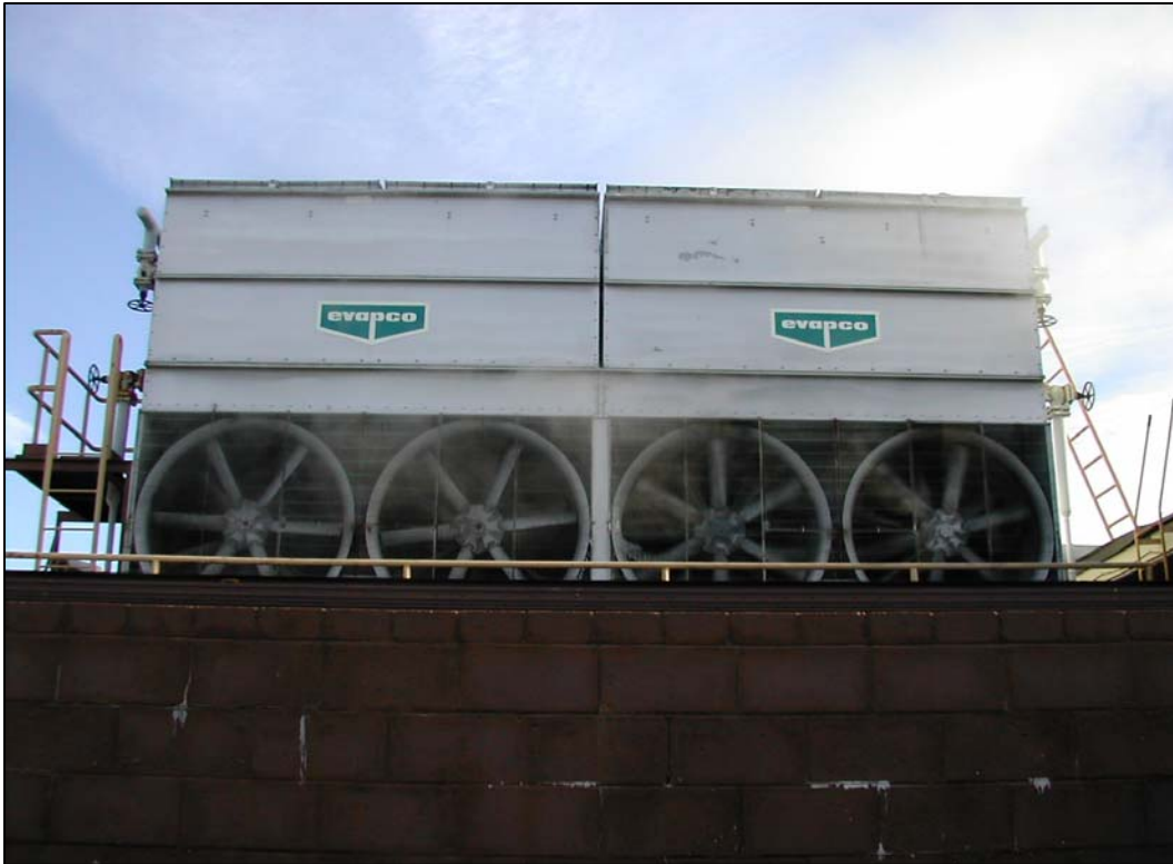
Figure 1 – Cooling Tower Before.
