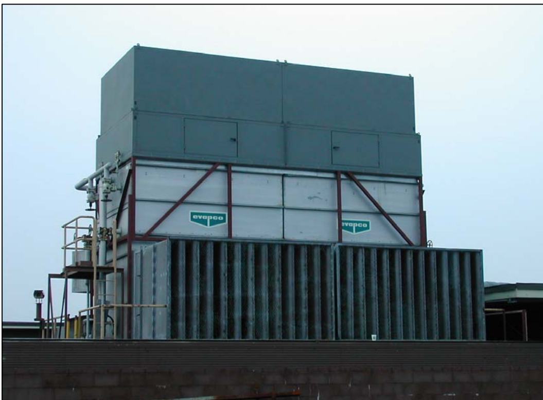
Figure 2 – Cooling Tower After.
